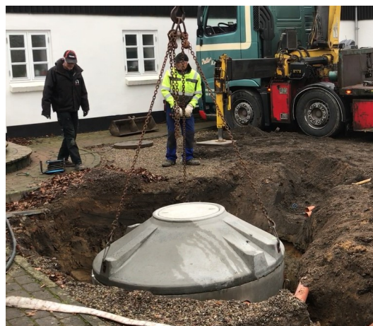
BioKube Betong installeras
